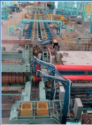
Flat Steel Production Line
