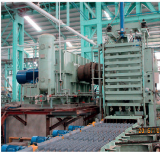
Split 650T Cold Shear
