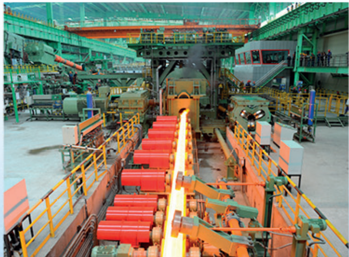
Seamless Pipe Production Line
